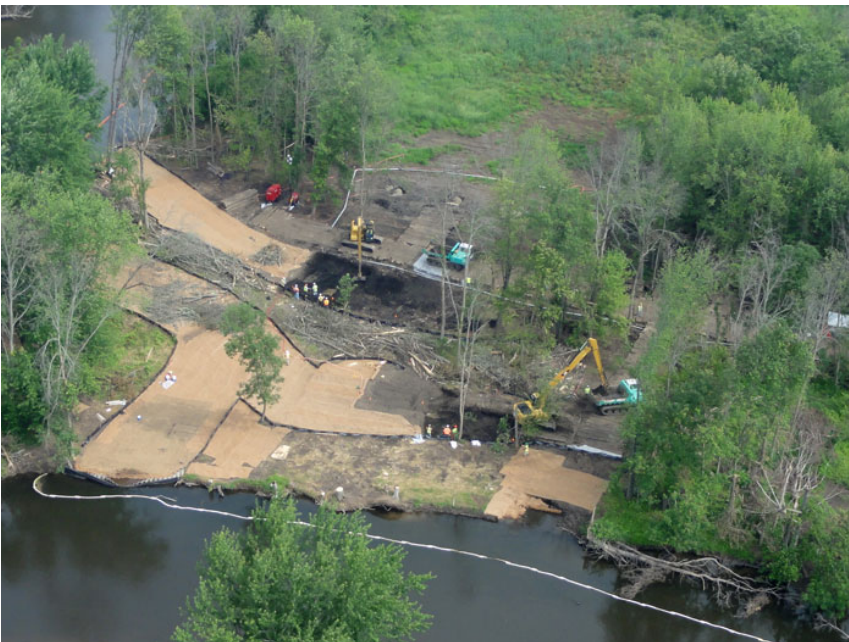
Overbank excavation at mile post 11.25 (7/18/2011) (EPA)
