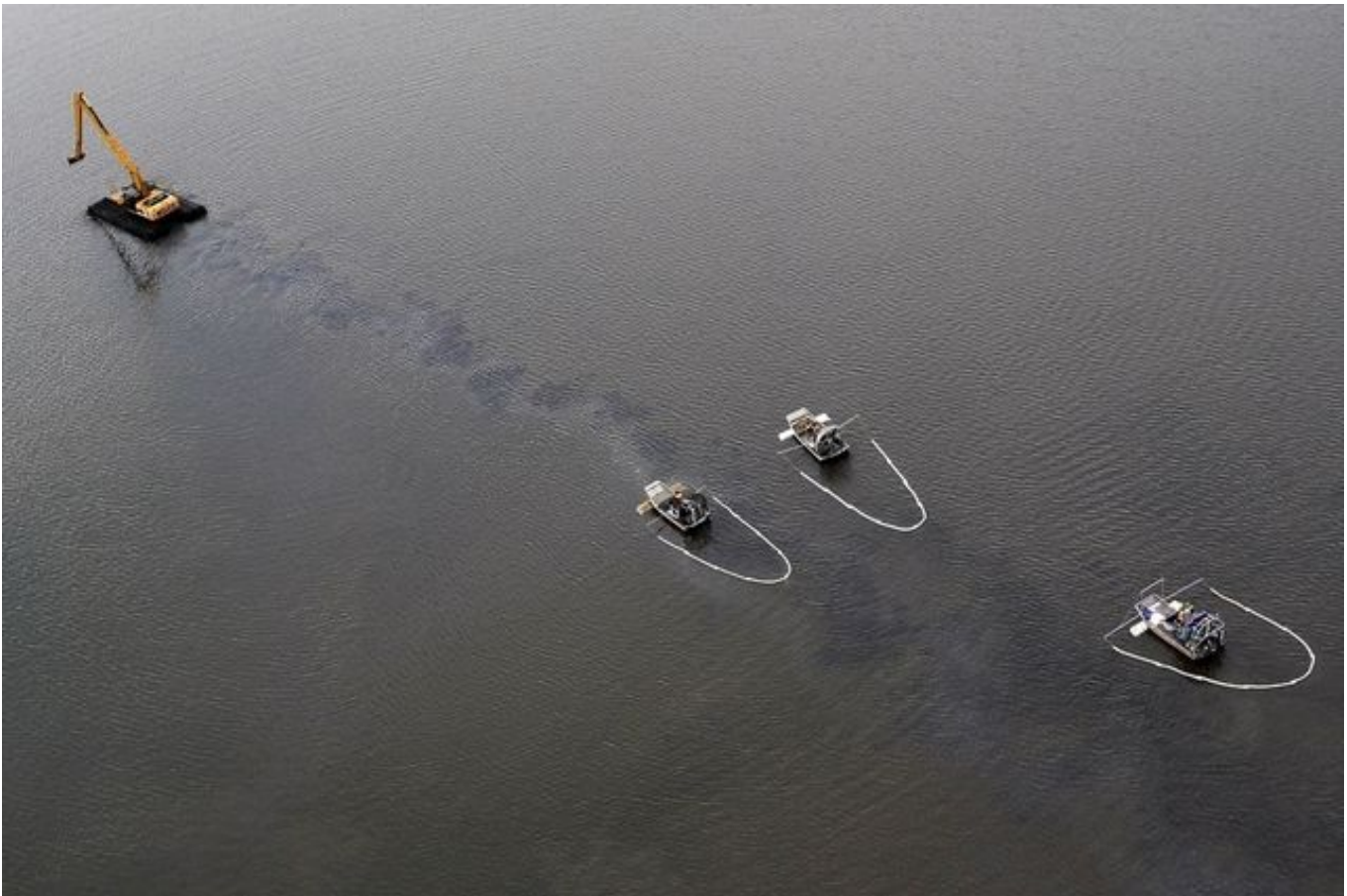
A pontoon boat stirs up submerged oil and three sheen sweepers collect the oil that is stirred up. Photograph by John Grap/The Enquirer/AP Photo http://www.bloomberg.com/slideshow/2012-07-25/enbridge-s-quiet-765-million-oil-spill.html#slide18
